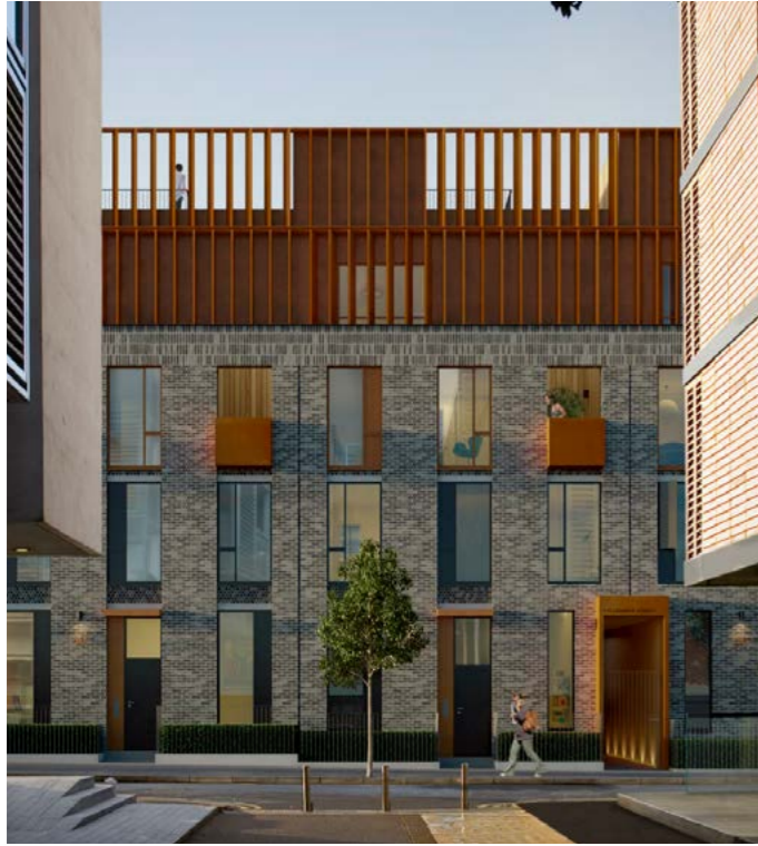
Roof Gardens, Manchester. Weathering steel is used to add colour to the facade and a nod to the industrial context.
