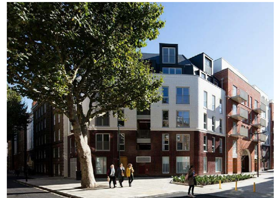
Bourne Estate regeneration, London. A varied street scene with variety in materials and massing enlivens the street.
