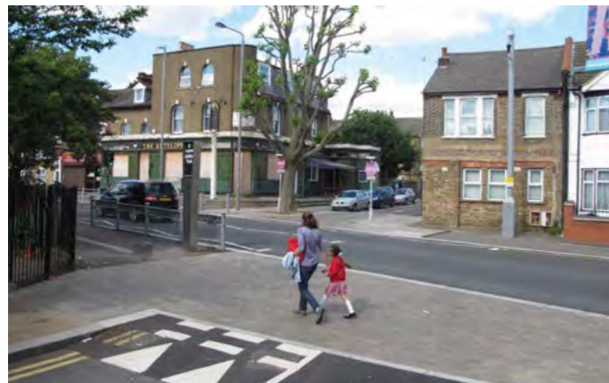
Example of continuous footway
