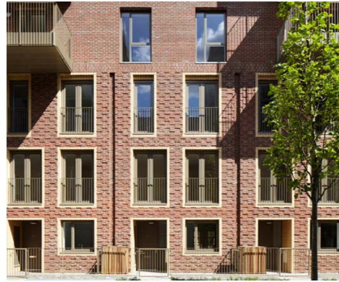
St John's Hill Peabody Estate, London. Frontages incorporate entrances for individual homes as well as communal entrances.
