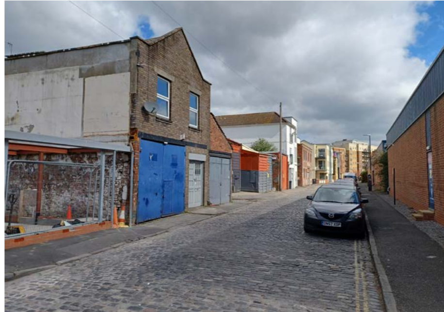
Stillhouse Lane as existing
