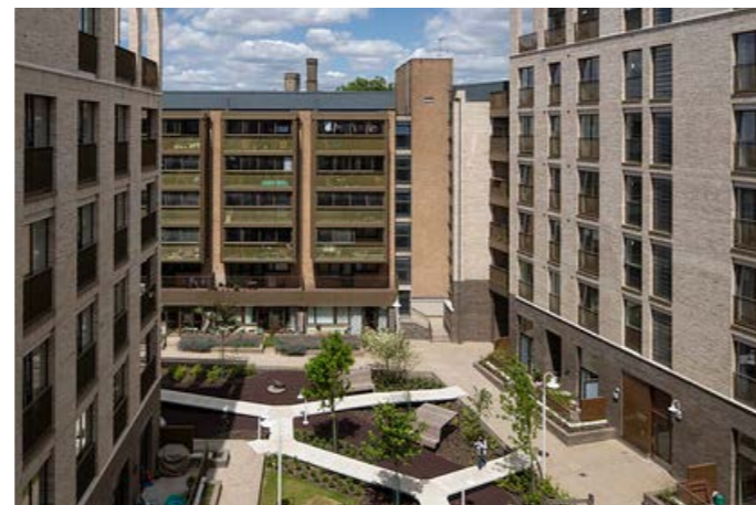
Kings Crescent Estate, London. Mid-rise buildings can provide dense development while retaining a human scale on the street.
