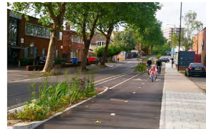
Existing Whitehouse Street cycle track.
