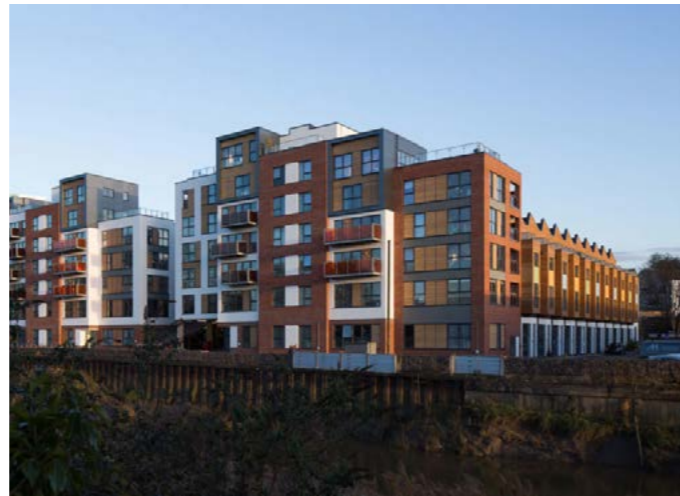
Paintworks Phase III, Bristol. This development provides relatively high density for the inner urban area with a mix of low and medium rise homes and workplace.
