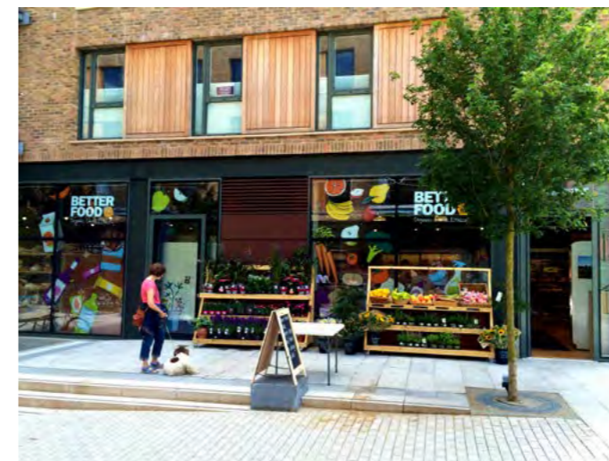
Gaol Ferry Steps, Bristol. The active frontages enliven the street and the buildings provide a desirable sense of enclosure.
