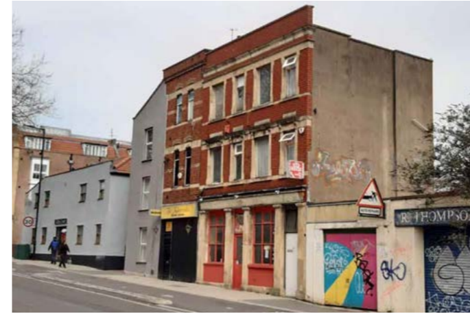
Existing Whitehouse Street frontages
