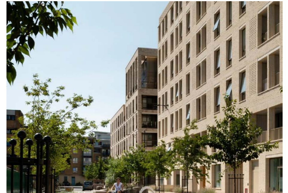
Precedent: Medium rise residential development in the King's Crescent Estate, London. New street trees line the new frontage.
