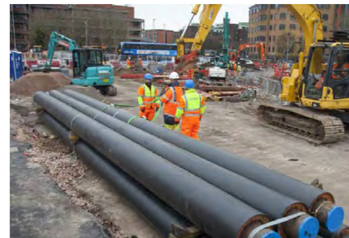
Installation of Redcliffe heat network
