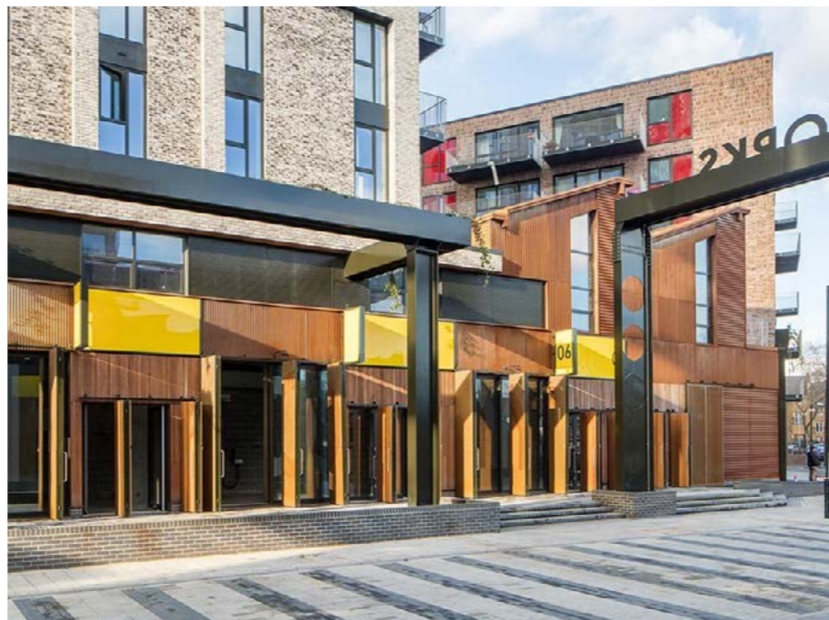
Caxton Works is a mixed-use development in Canning Town in east London which provides flexible and affordable light industrial /workshop units with homes above.
